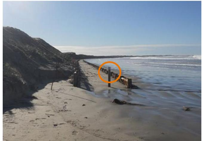
Figure 2: Wet-sand fencing at Port Fairy, June 2014. Fence was installed in March, 2014.
